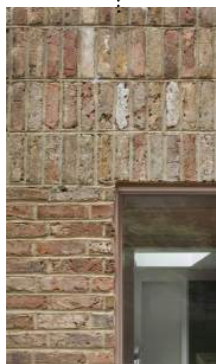
Vertical stack bond / soldier course brick banding
