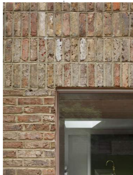
Vertical stack bond / soldier course brick banding
