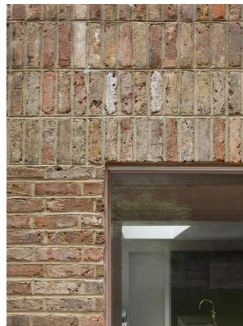
01 Vertical stack bond / soldier course brick banding
