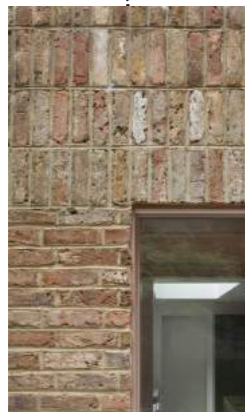
Vertical stack bond / soldier course brick banding
