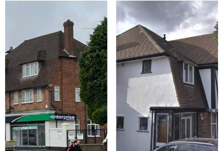
Roof profiles of 239 and 245 Watford Road with the roof enclosing an additional storey on the street facing elevation than on the flank elevation
