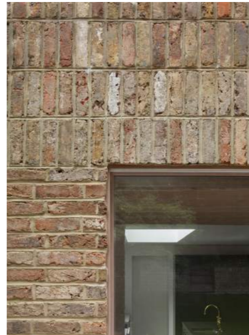
01 Vertical stack bond / soldier course brick banding
