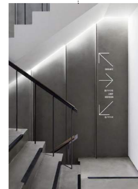
Integrated signage and stair
