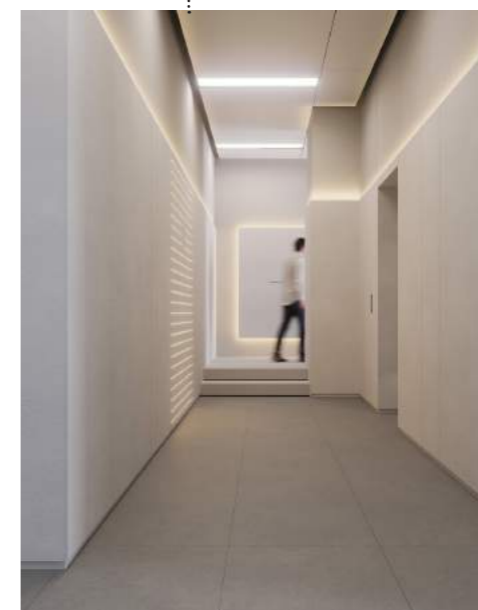
Dropped ceiling with integrated lights
