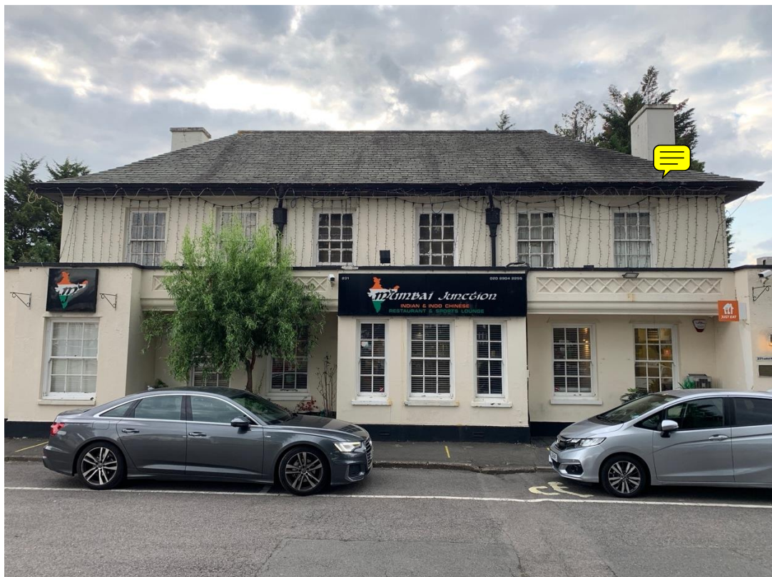
Fig 2: 231 Watford Road from E.
